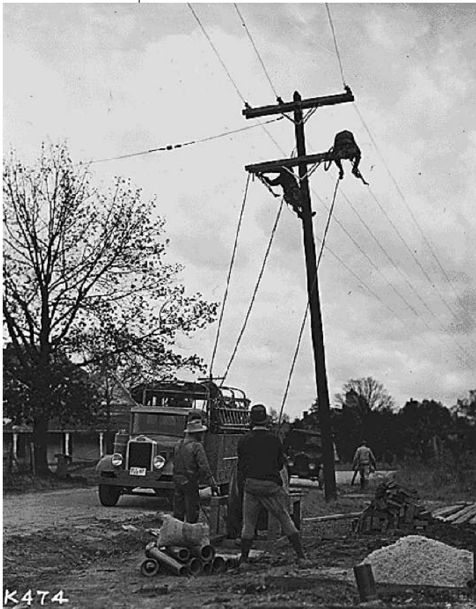
Stringing a rural electricity transmission line during the 1930s.
